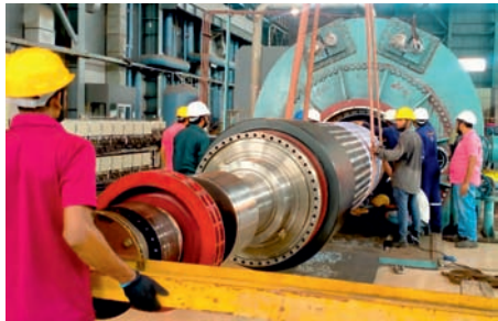
Major Overhauling of 300 MW LP Turbine & 135 MW Generator
